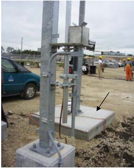
Photo 4-4: Example of a slab on grade foundation
